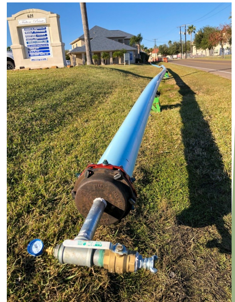
Pipeline is laid out along Fulton Beach Road in preparation for the relocation of utilities to Key Allegro.
