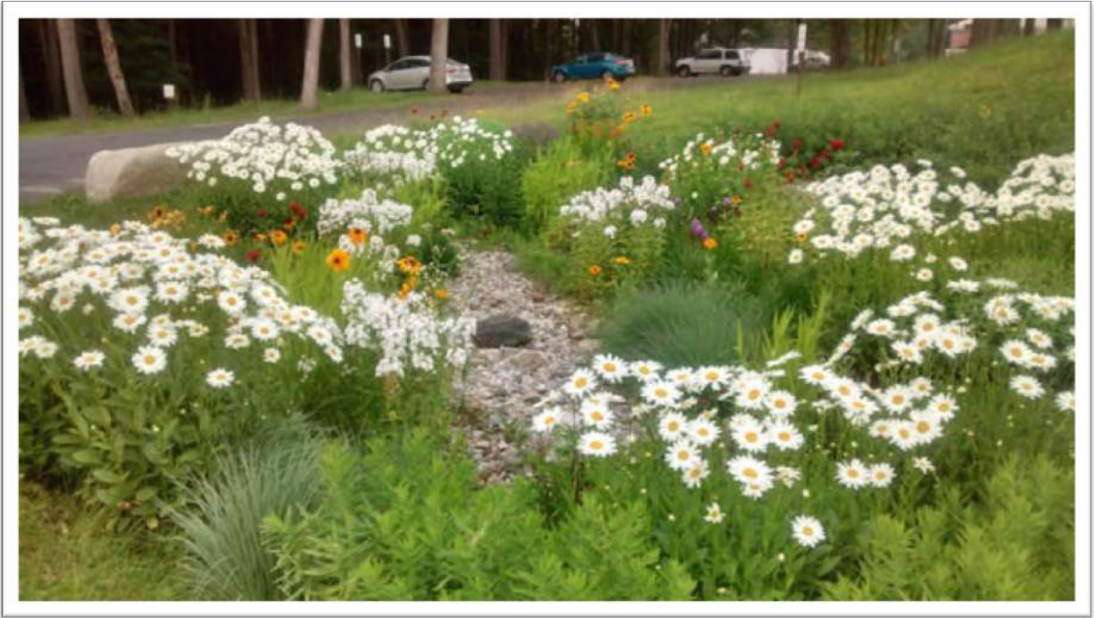
Figure 4: An example of a rain garden designed to capture runoff from a nearby parking lot. Source: US Environmental Protection Agency.
